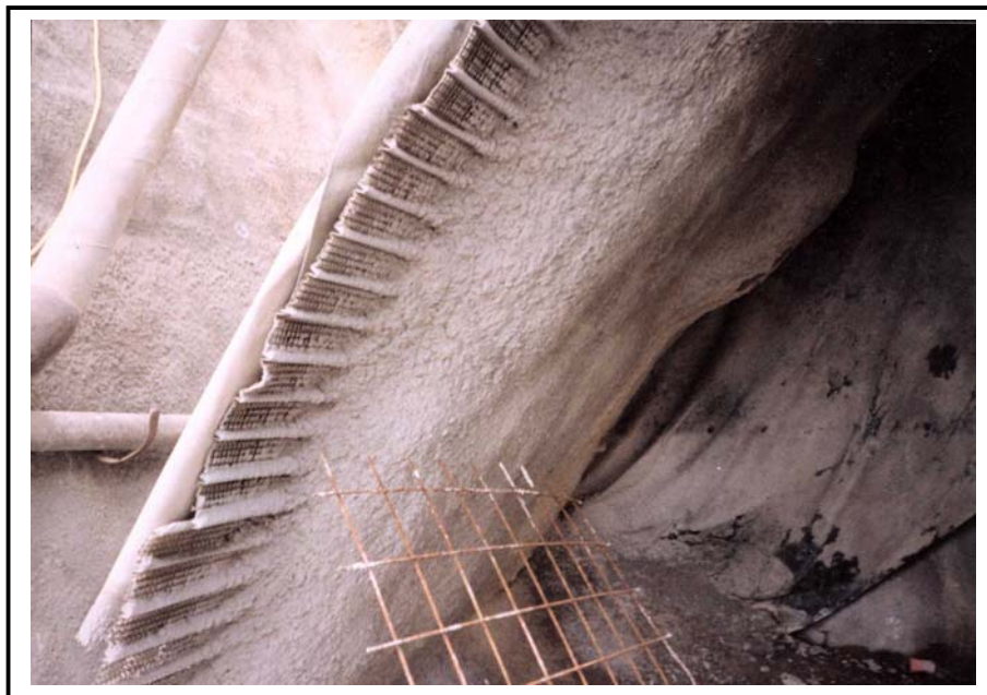
Fig. 20 Sprayed concrete to shell structure
