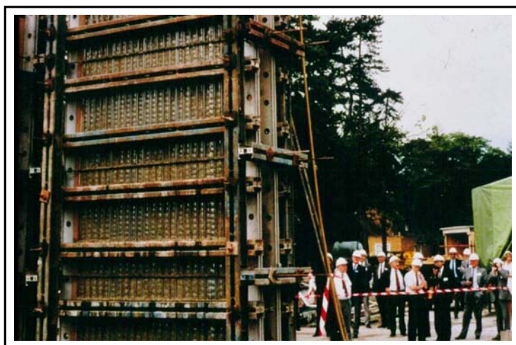
Fig. 24 View of BCA Hy-Rib 5m Wall Trials
