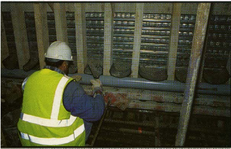
Scraping away excess material during pouring
