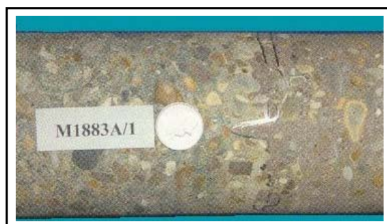
Fig 26 View of core at Hy-Rib lap position Panel 3 / 5
