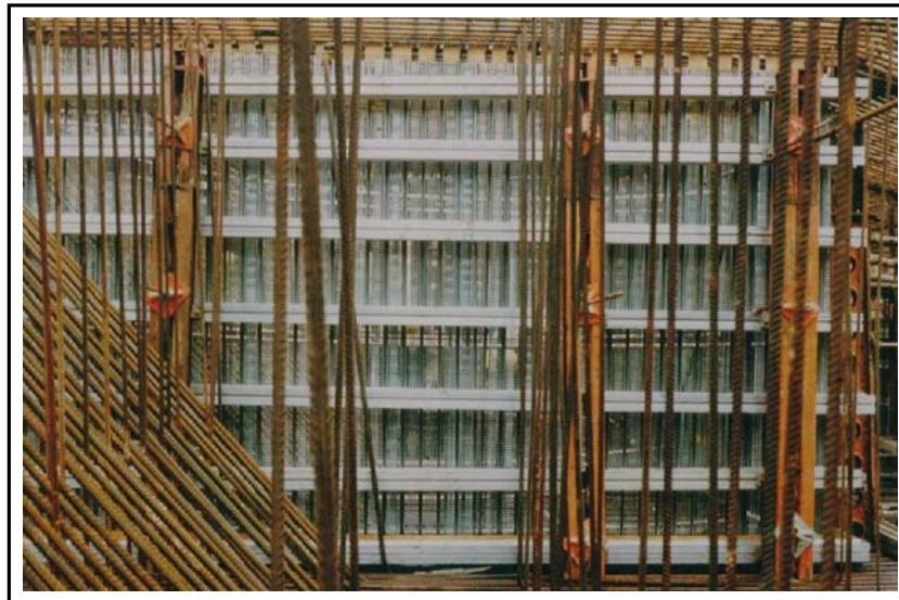
Fig. 10 Application of Hy-Rib to 3m deep stop end.
