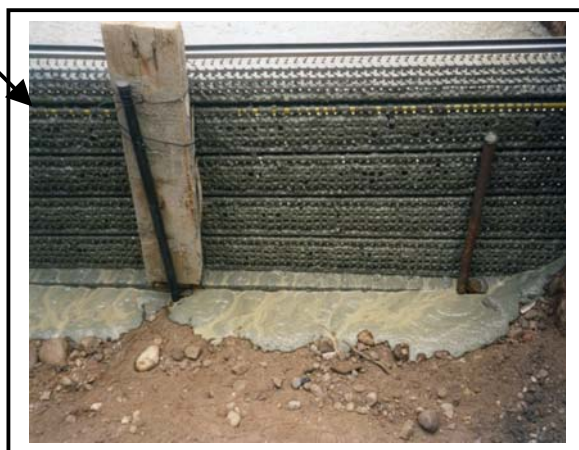
Fig 6 View of 360 deep stop end with self compacting concrete
